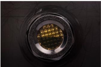
11. If the glass is half darkened, there is still a capacity of approx. 1.3 litres. If it is completely darkened, the tank must be emptied.
